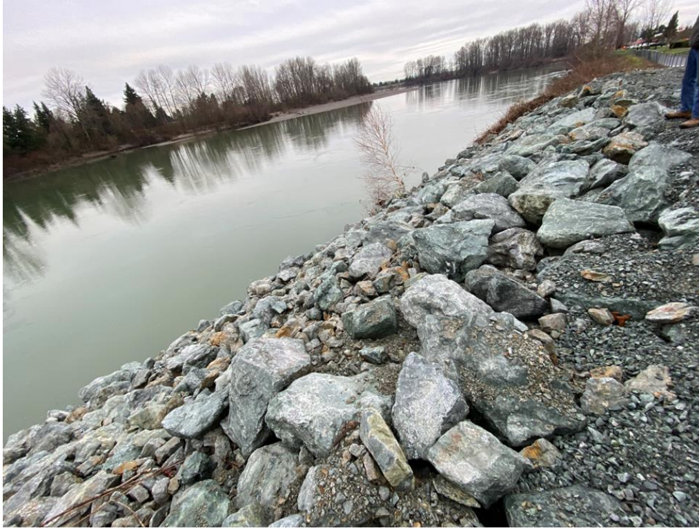
Photograph 5. Site visit to DD 3 levee on the Skagit River in February 2022 depicting emergency flood repairs completed in November 2021 immediately following a flood event.
