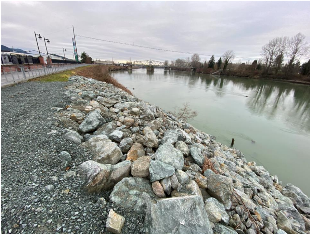
Photograph 6. Site visit to DD 3 levee on the Skagit River in February 2022 depicting emergency flood repairs which were completed in November 2021 immediately following a flood event.
