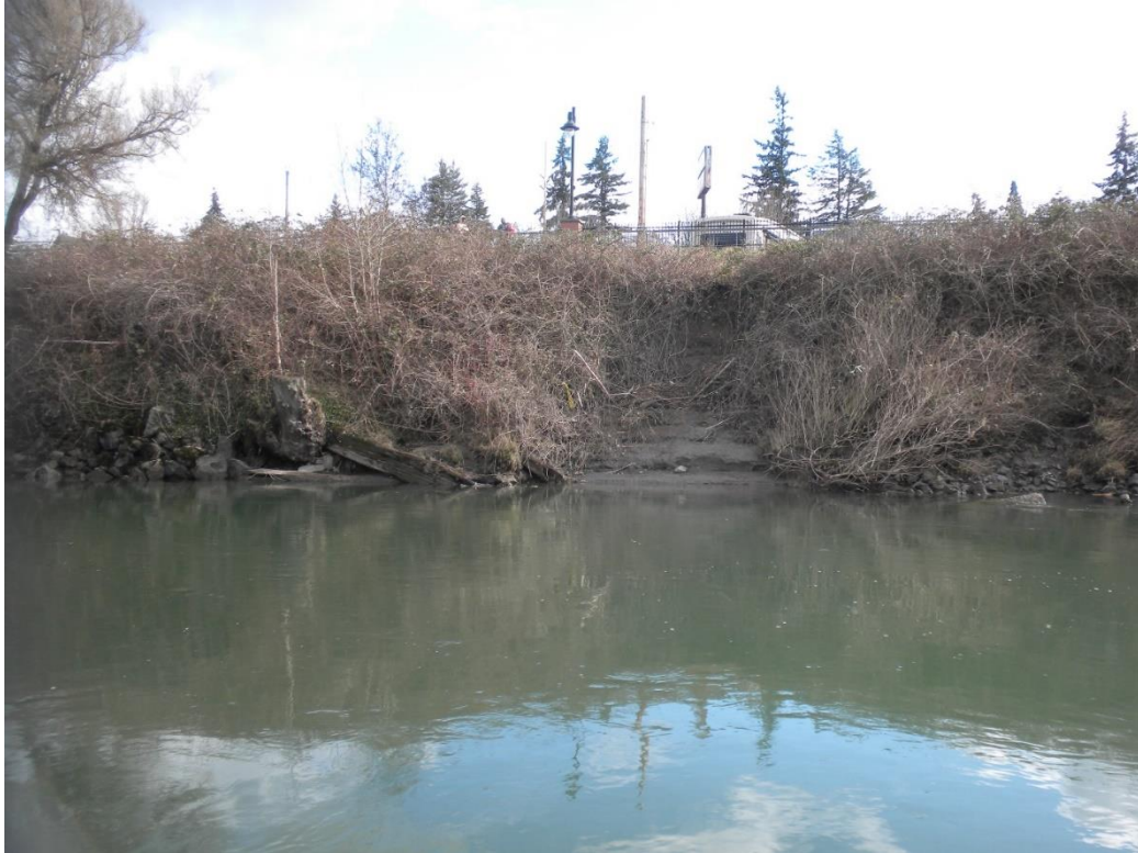
Photograph 3. DD 3 levee repair site on the Skagit River showing slope failure from 2020 flood event.
