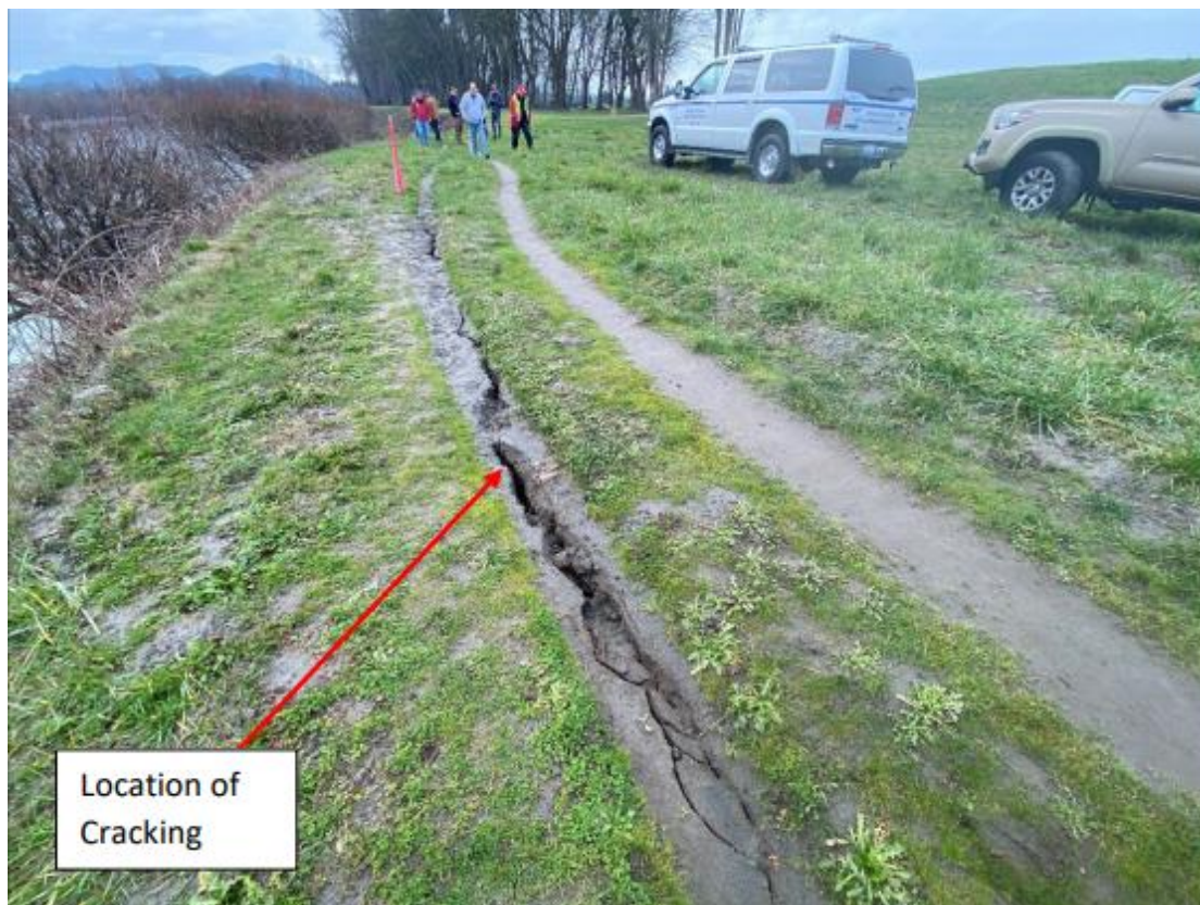
Photograph 11. Location of the cracking on DD 12 site 3 oriented downstream.
