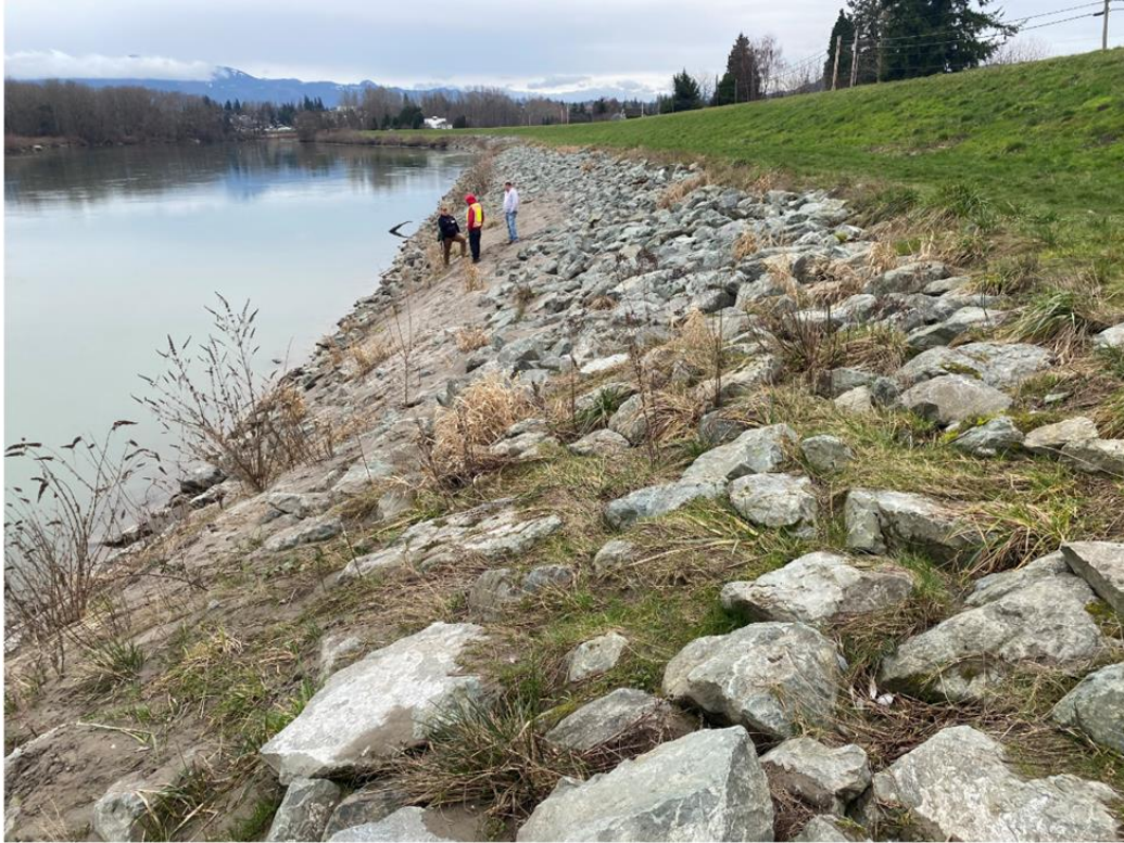
Photograph 1. Site visit to DD 1 levee on the Skagit River in February 2022 depicting scoured slope because of the November 2021 flood event.
