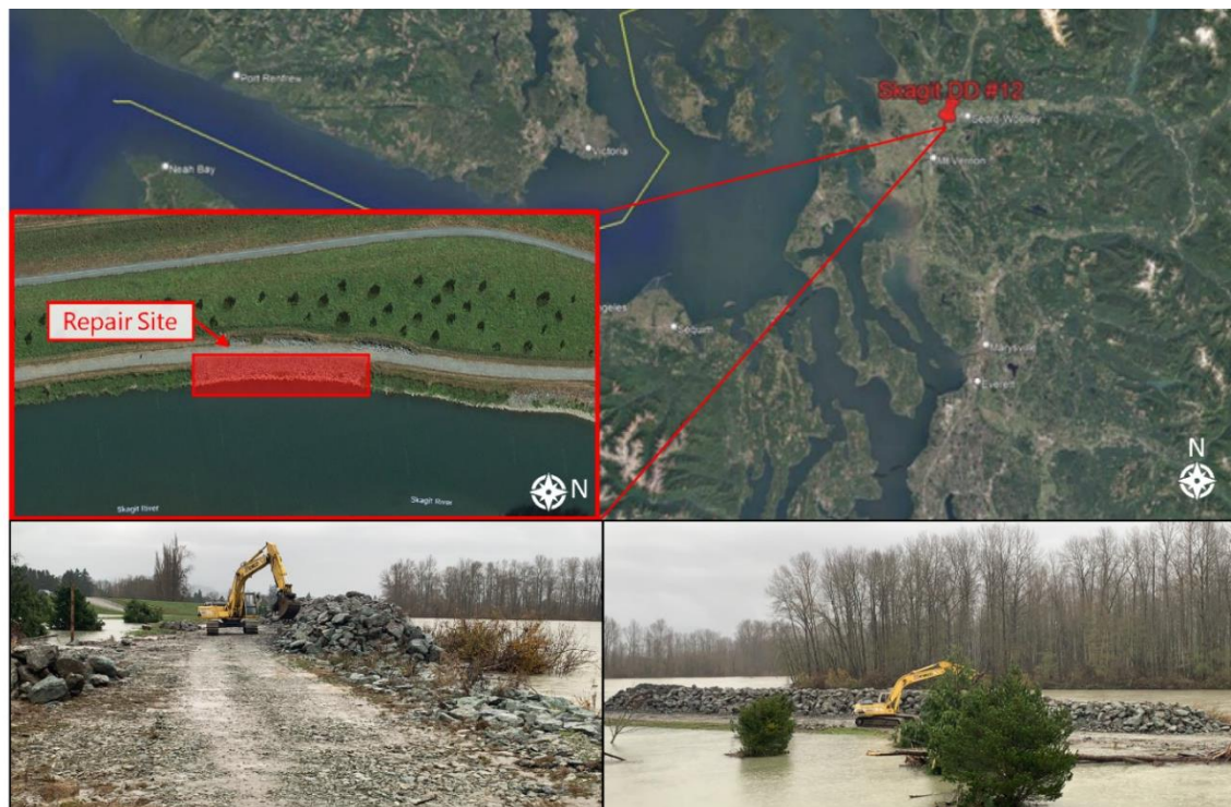
Photograph 9. Photos and map showing extent of the flood fight activities at the DD 12 Site 1 levee repair during the November 2021 flood event in the Skagit River. No in-water work occurred. Rock was stacked on top of rock previously placed during the February 2020 work along the bank and above the waterline of the river during the flood. The bottom two photos show the addition of rock in 2021.
