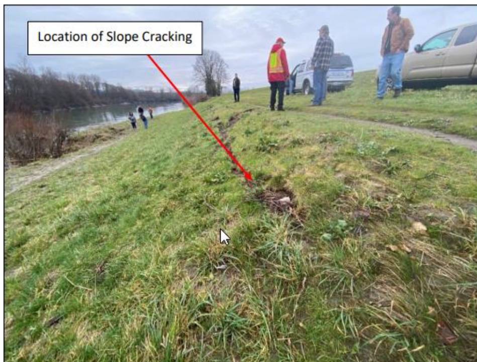
Photograph 10. Location of the cracking on DD 12 site 2 oriented downstream.
