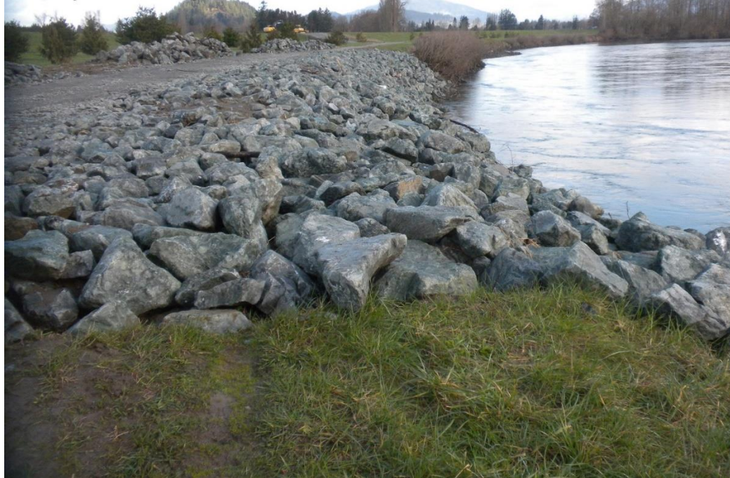
Photograph 8. Emergency repair work completed in February 2020 along 300 LF of DD 12 Site 1 on the Skagit River. The photograph is looking upstream.
