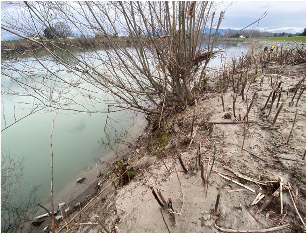
Photograph 2. Site visit to DD 1 levee on the Skagit River in February 2022 depicting scoured slope because of the November 2021 flood event.
