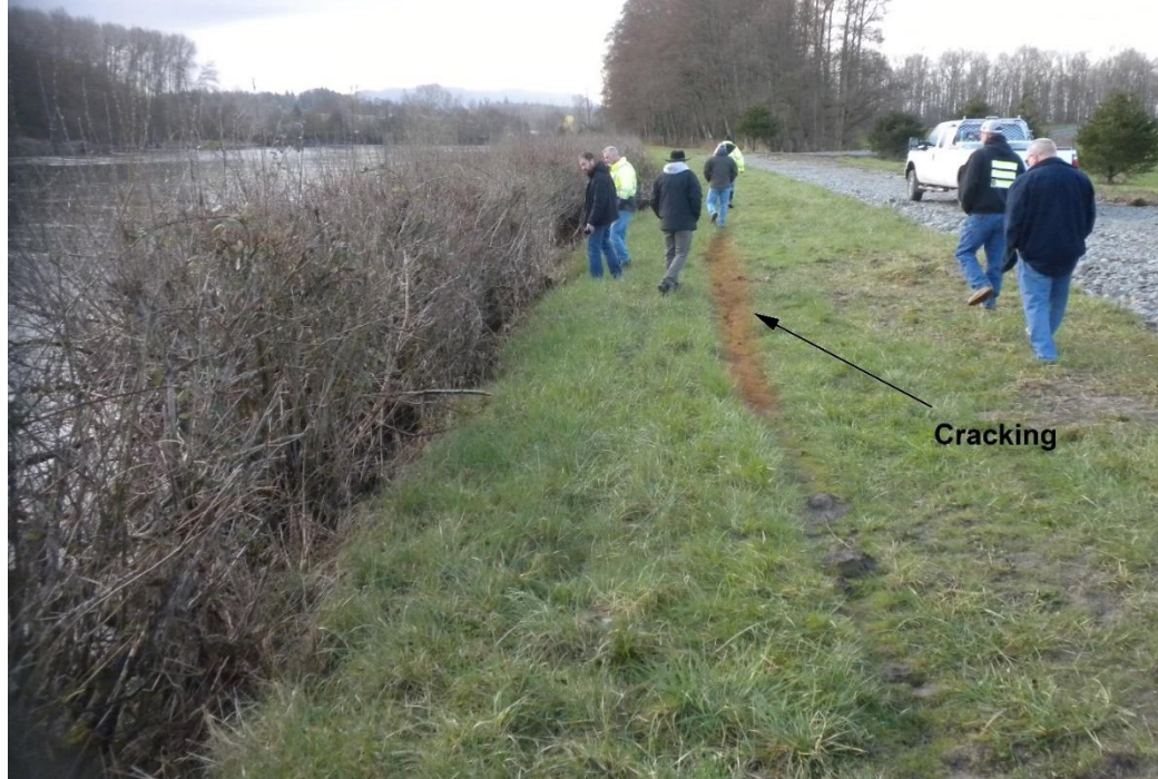
Photograph 7. Additional cracking observed along the riverward bench of DD 12 Levee Site 1 on the Skagit River in March 2020 after February 2020 flood event.
