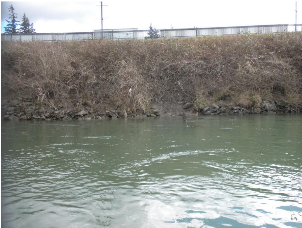
Photograph 4 Scour at damaged segment of DD 3 levee on the Skagit River following 2020 flood event.
